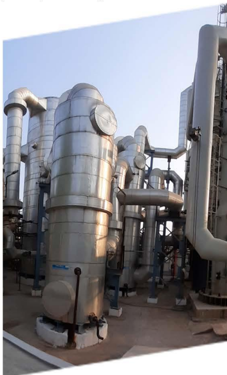
2000 TPD Sulphuric Acid Plant, IFFCO Paradeep Unit, Paradeep Construction nearing Completion
